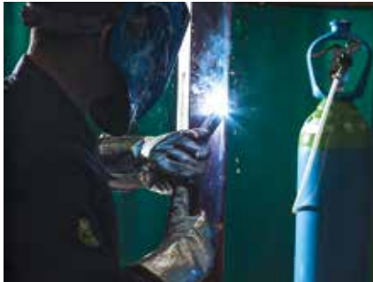
MAG welding of carbon steel
