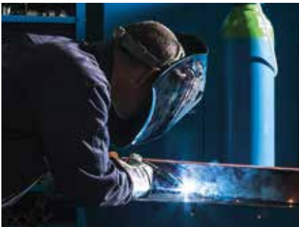
Manual MAG welding
